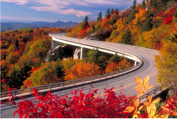
Linn Cove Viaduct crosses Grandfather Mountain.
